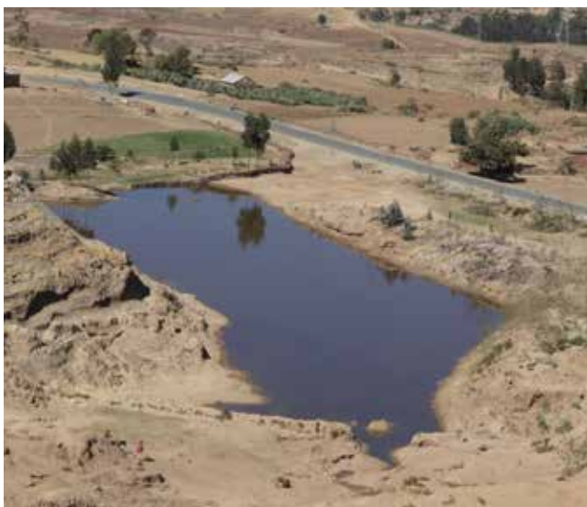
Figure 37: A borrow pit connected to a road acts as a small earth dam. Photo: MetaMeta.
