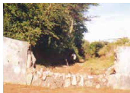
Stage 3: Spillway is raised to 50 cm above new sand level
