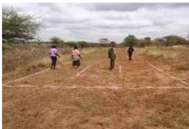
Figure 13: Farm pond layout and excavation. Photos: S. Ngigi.
