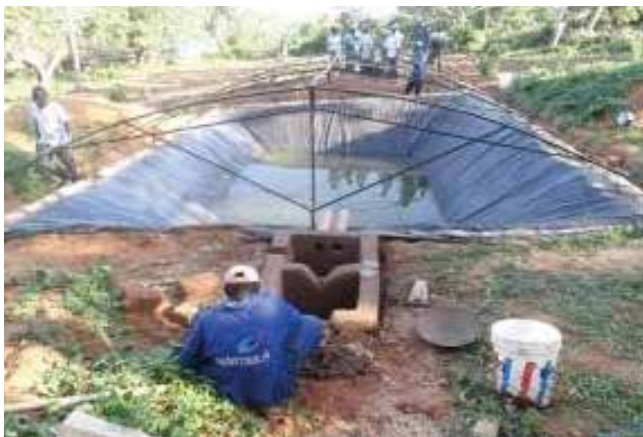
Figure 15: Farm pond roofing process. Photos: S. Ngigi.
