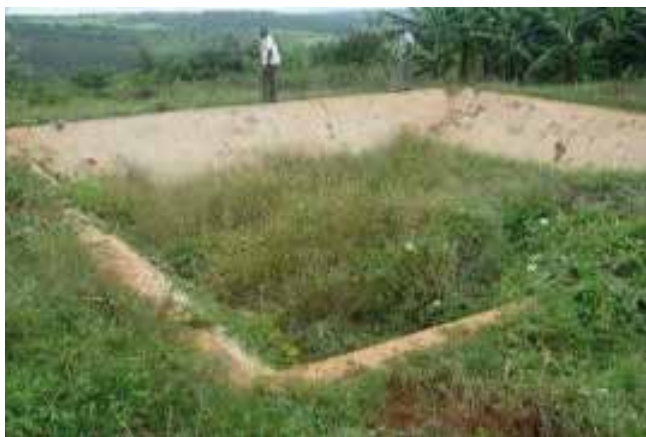
Figure 7: On-farm ponds affected by siltation, evaporation and seepage. Photos: S. Ngigi.
