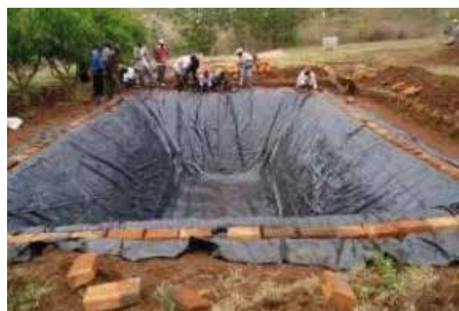
Figure 14: Lining the farm pond including masonry layer for anchoring the dam liner. Photos: S. Ngigi.
