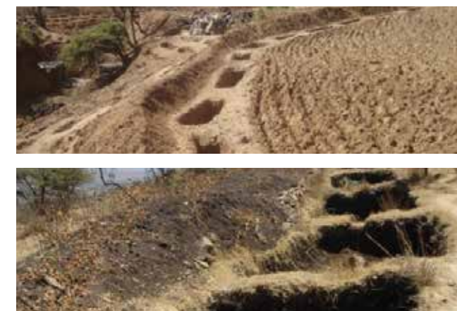
Figure 56: Infiltration trenches (left) and a percolation pond (right) in Ethiopia. Photos: K. Woldearegay and MetaMeta.
