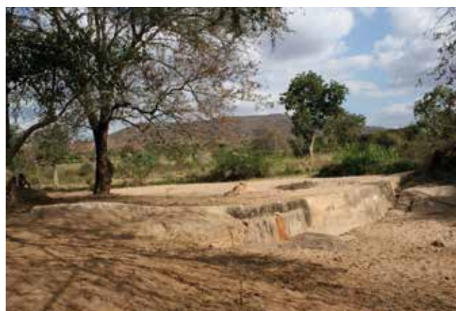
Figure 23: The increase in sand sediments on the original riverbed caused by the construction of a sand storage dam: a diagram (left) and a real-life example (right). Source: Pixinit Studios. Photo: J. de Trinchieria.
