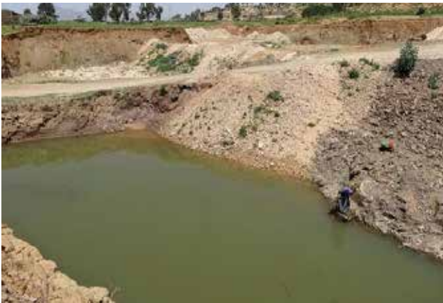
Figure 40: A borrow pit made from the excavated soil of a road construction. Photo: MetaMeta.
