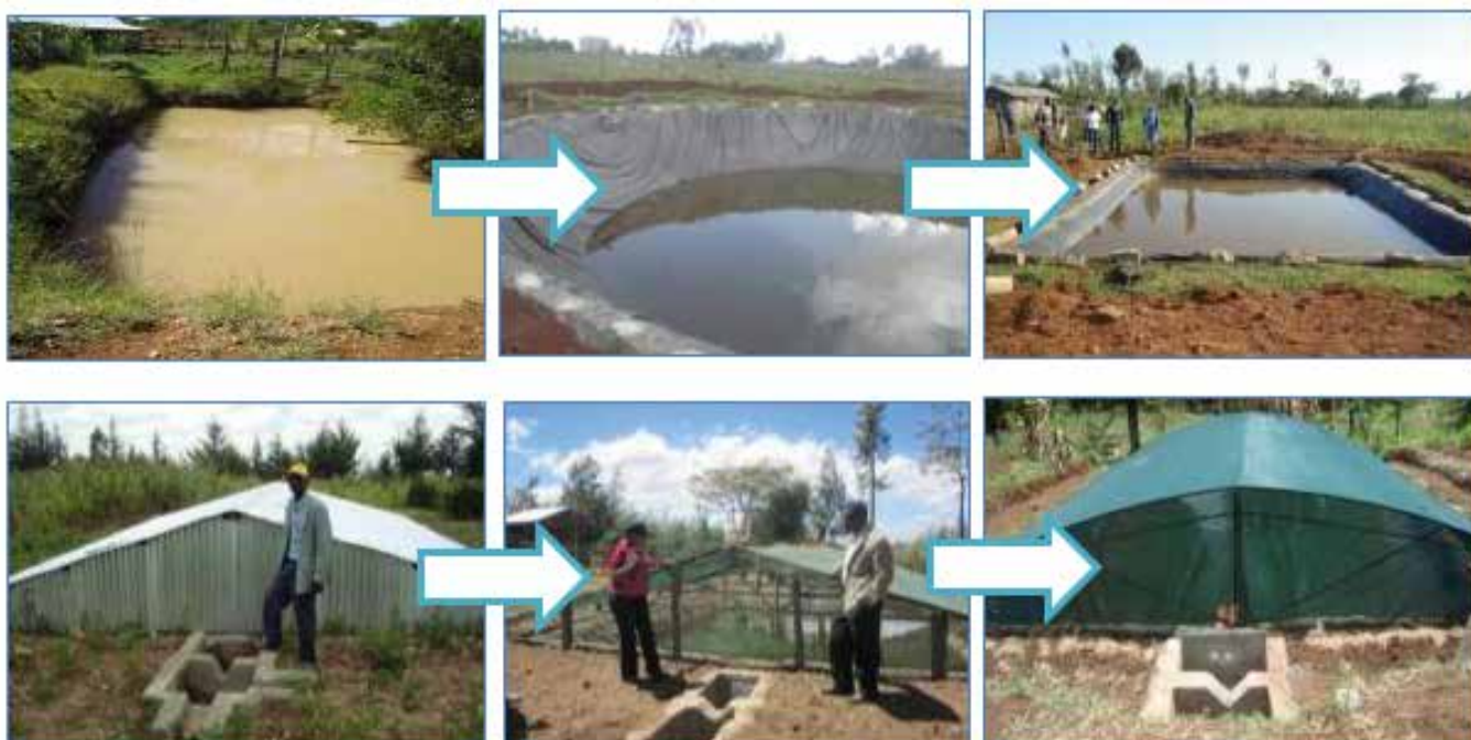
Figure 8: Evolution of control measures for seepage and evaporation water losses. Photos: S. Ngigi.
