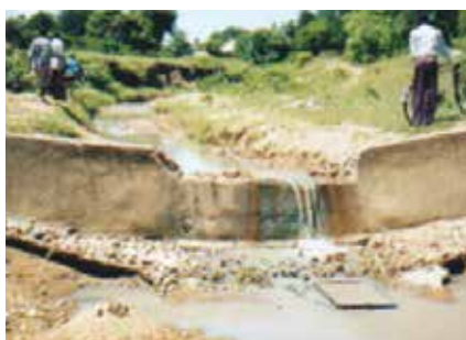
Stage 5: Spillway is raised to 50 cm above new sand level.
