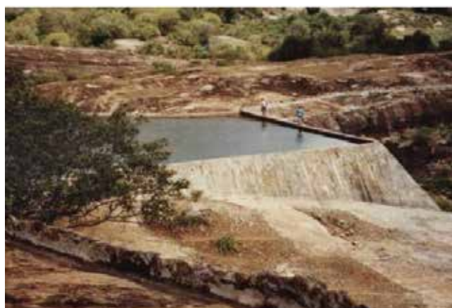
Figure 49: A rock catchment with a tank (left) and a dam on the rock itself (right). Photos: J. de Trincheria and E. Nissen-Petersen.
